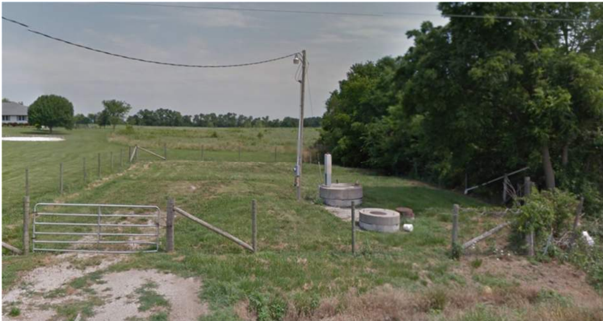
Figure 2.3 -- Northeast Lift Station
