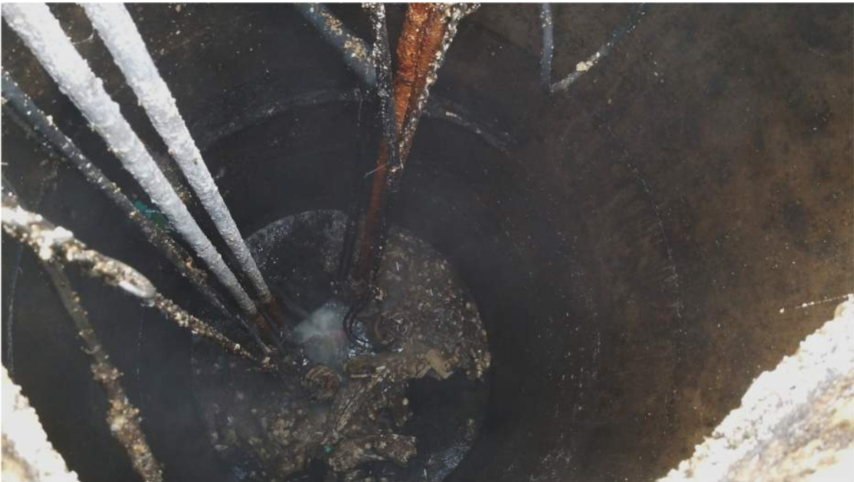
Figure 4.4 -- Northeast Lift Station Interior
