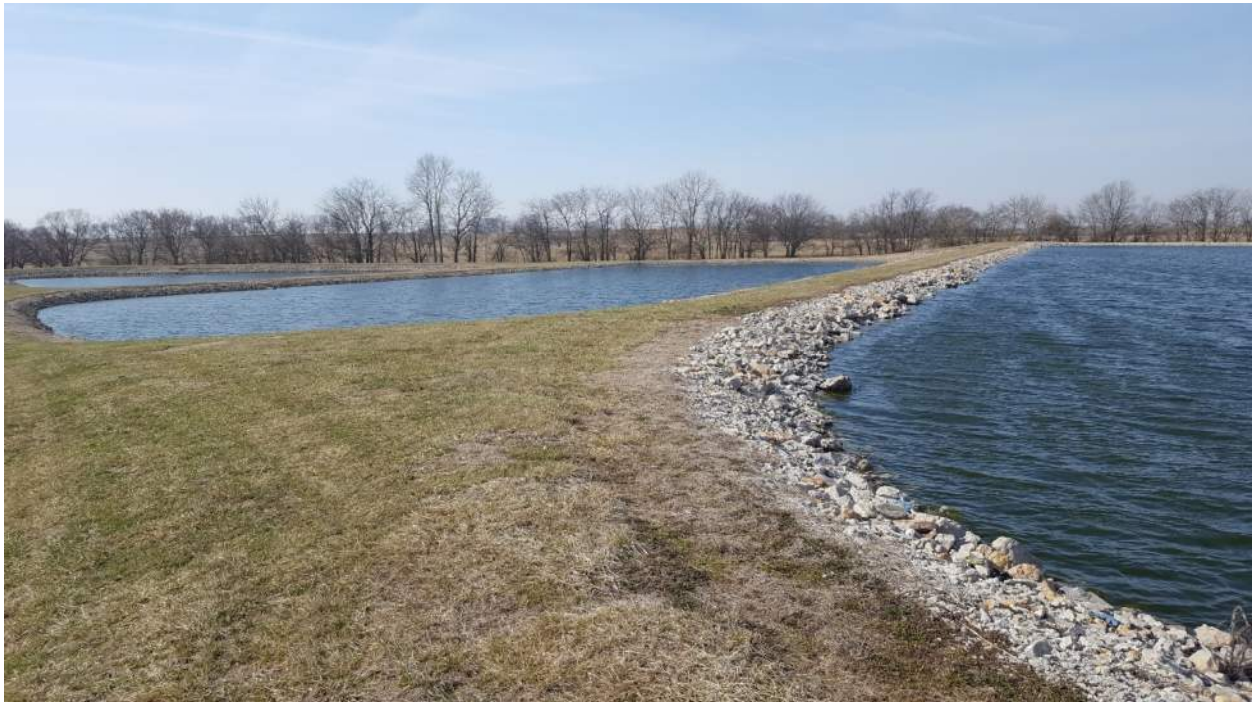
Figure 2.5 -- Lagoon Cells Looking Southwest
