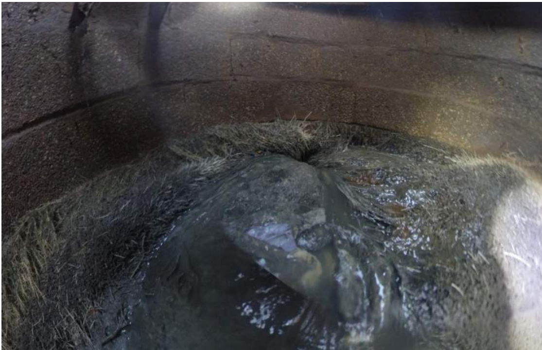
Figure 4.3 -- Manhole 3 Roots
